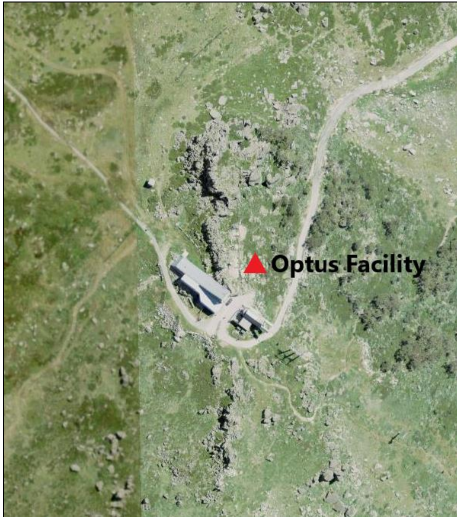
Figure 1: Existing Optus facility
